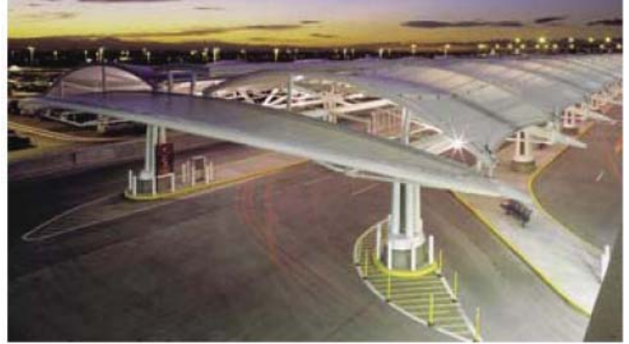
Como Park Visitor and Education Resource Center, Merit Award, I.D.E.A.S. Awards sponsored by AISC, Hammel, Green and Abrahamson, Architects and Engineers
